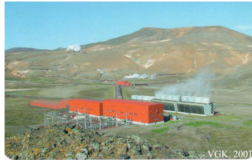
A geothermal power plant
