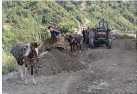
Sand Dumping on Road Side near confluence of Poonch River and Bann Nullah
