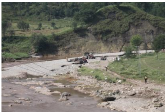
Sand and Gravel Extraction at Khuairatta
